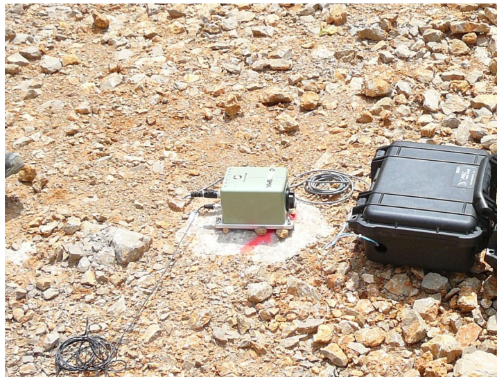
Figure ESM02-1. Nanometrics TitanSMA accelerograph installed directly over a rock outcrop.
