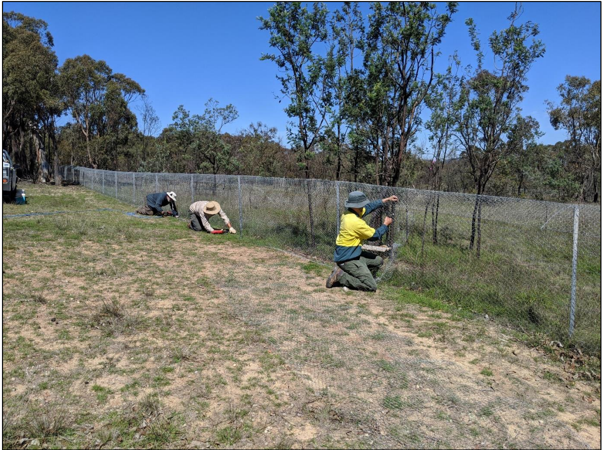
Fig. 3 Volunteers and Parks and Conservation Service Rangers constructing the retrofitted Mini Safe Haven (MSH) fence with floppy top and 35 x 25 mm aperture wire mesh (permeable to mice) secured over the pre-existing larger mesh. The fence footing was more easily pinned flush to the ground when grass was cut short before construction. We recommend constructing MSHs away from drainage lines and soggy soil, and suggest the footing be covered in gravel or buried vertically to reduce maintenance effort. Gravel may be more suitable where corrosive soils would damage the fence. Refer to the main text for an illustration with approximate measurements
