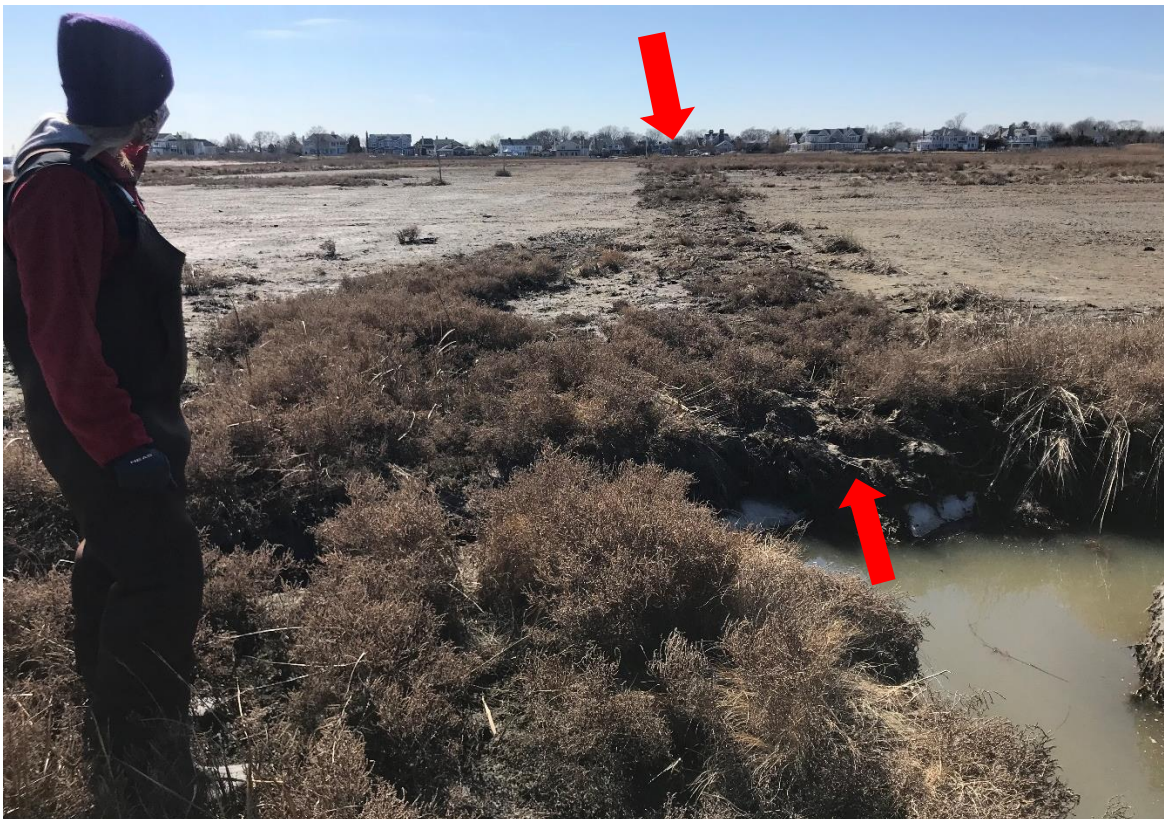
Suffolk County Photo 8. Gardiner Park West less than one-year post-restoration (03/08/21). Filled in linear mosquito ditch between the two red arrows. Aged coir log staked down and buried with peat collected from nearby micro-pool and runnel construction. Peat placed vegetation side up. Photo Nicole Maher @TNC
