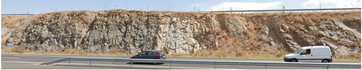
Fig. 24. Quarz-rich granite dykes in the Segovia's ring-road (Google Maps, Street View 2021)
