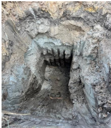
Fig. 1a: Open pit excavation
