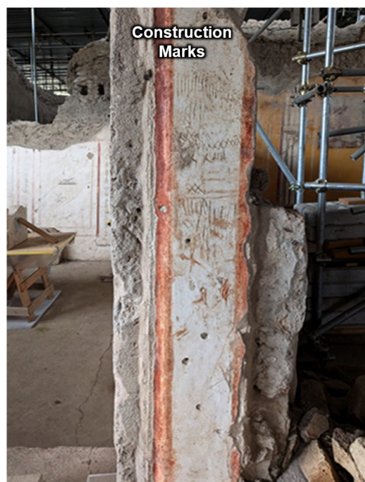
Supplementary Figure 2. Construction marks on walls in Room 2, including sequences of numerals and symbols.
