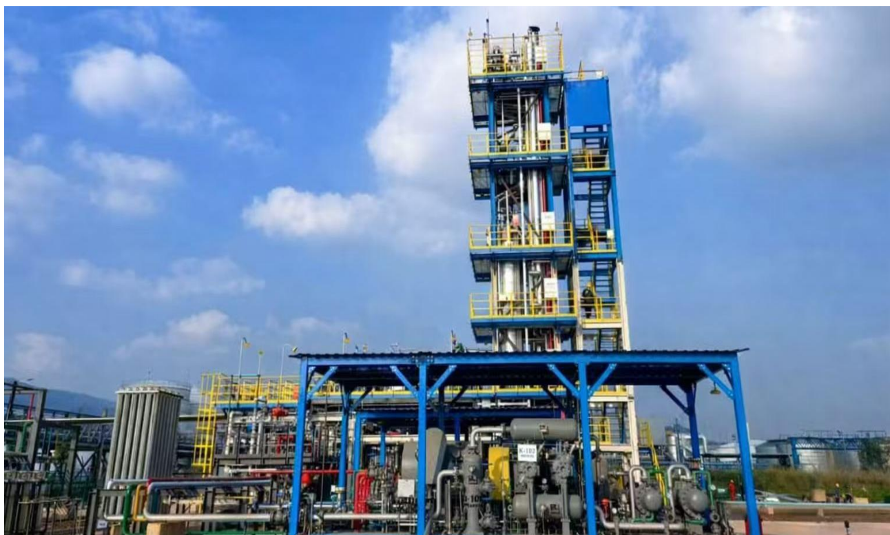
Supplementary Fig. 52 | Panoramic view of the 1000 tonnes/year FT-to-jet fuel production facility.
