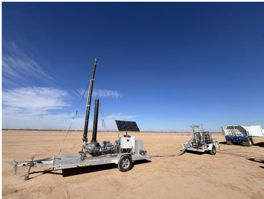
Figure S83. Photograph of the release stacks, pressure regulation unit, and CNG trailer
