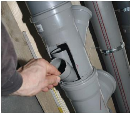
Figure 3: Moulding for the connection of the vacuum toilet
