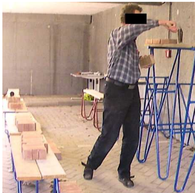
Figure 4. Laying bricks from a 45 cm support to 150 cm.
