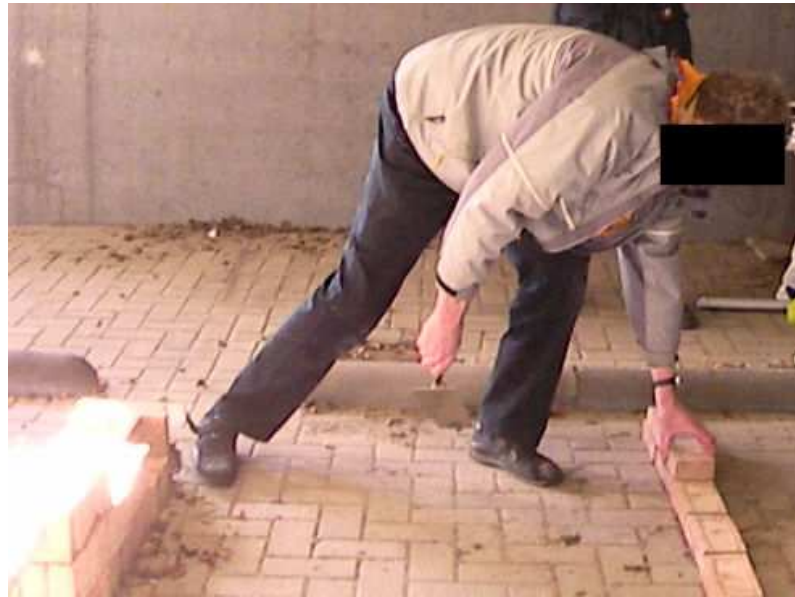
Figure 2. Laying bricks from ground to ground level.
