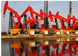
Oil-field Water Treatment
