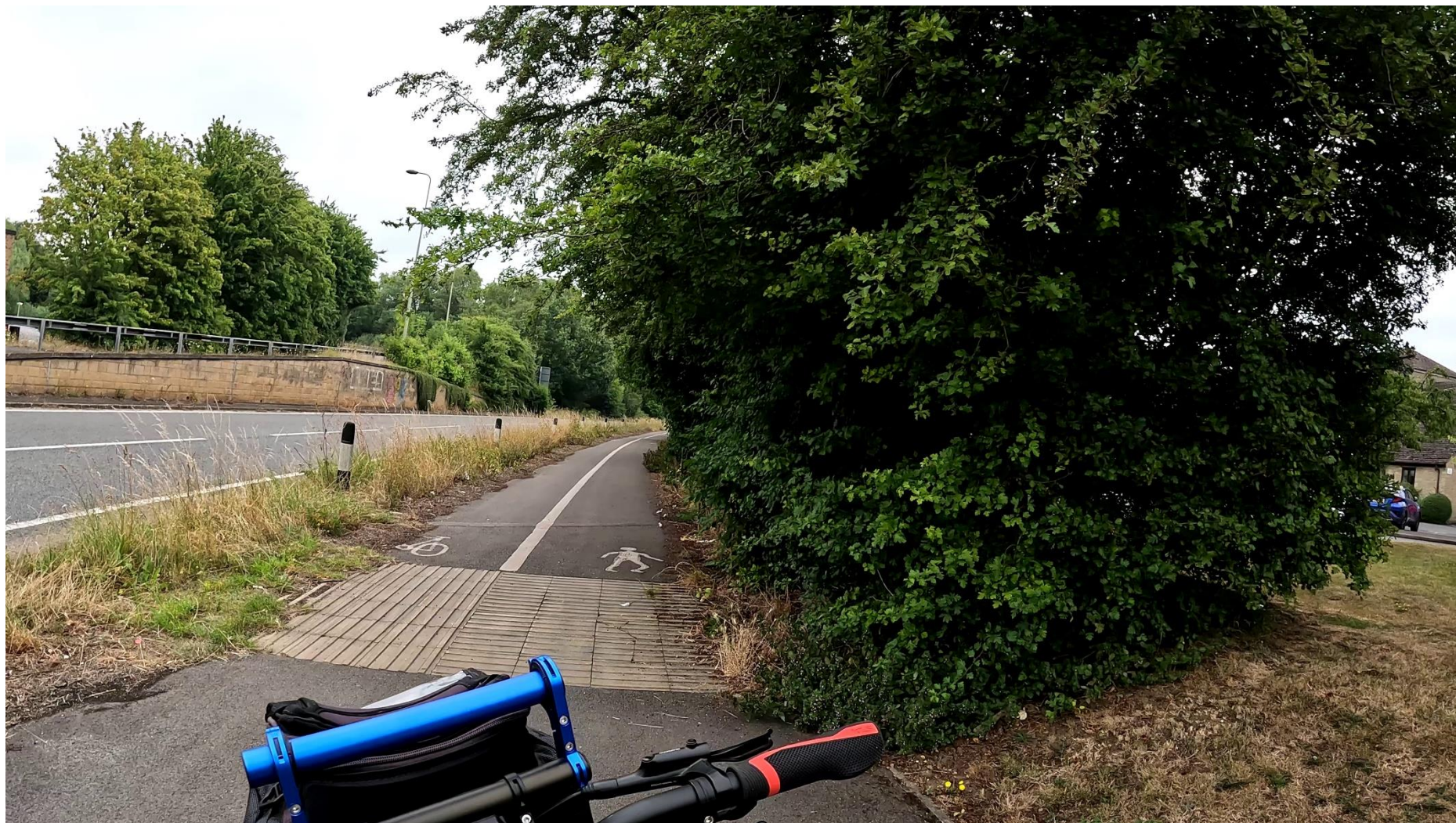
Picture 5: Overgrown shared path
