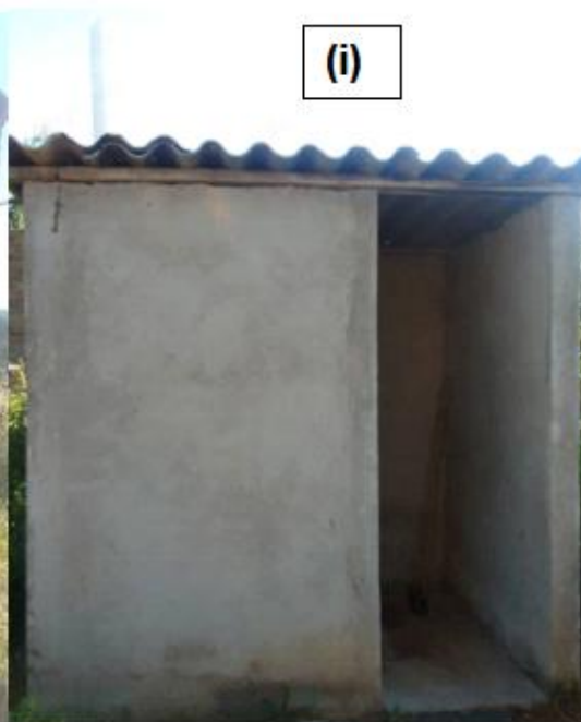
Completed BVIP latrine (Ward 1)
