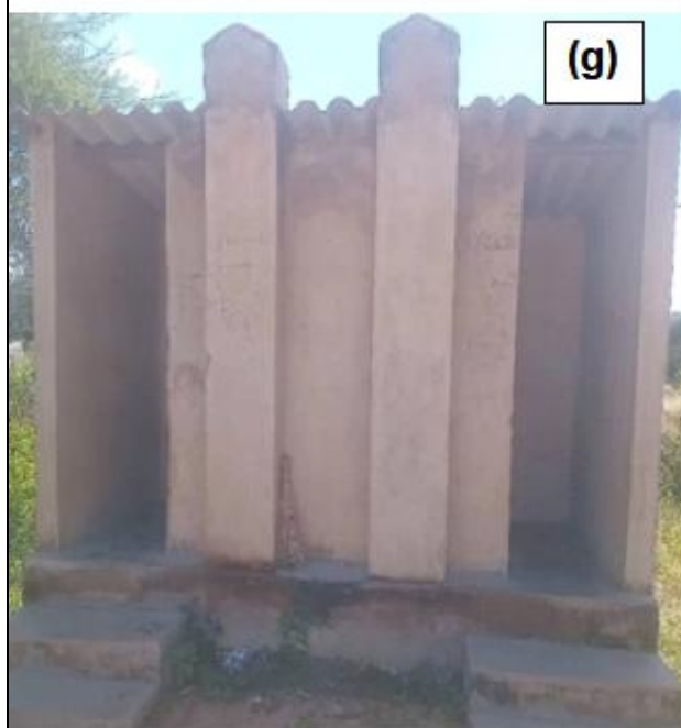
Completed dual conventional BVIP latrines (Ward 1)
