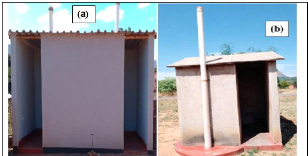
Completed dual conventional BVIP latrines (Ward 6) Conventional BVIP latrine design [17]
